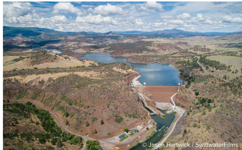
Iron Gate Dam
